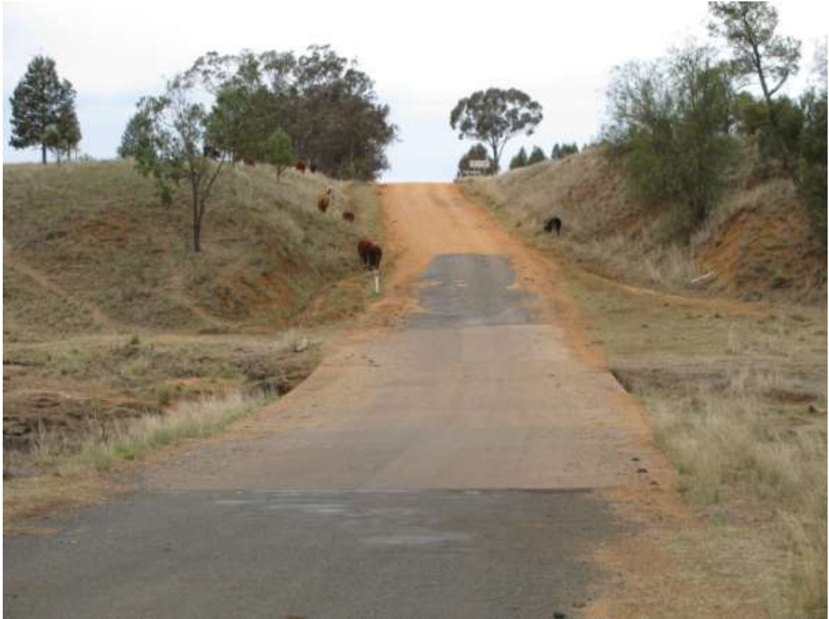
Photograph 1.0 - Saltwater Creek No 2 on MR129, looking east.
